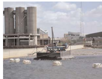
Sludge removal pontoon
